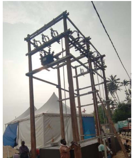
Standard plinth set up for installing multiple transformers.
